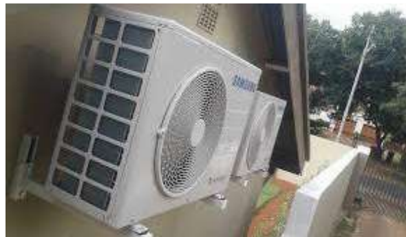
Installation of a 350 Hinged feeder pillar and residential aircons.
